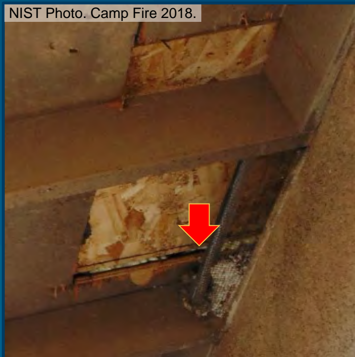
Failure: eaves/roof truss near eave vent
